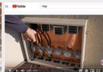
N6GR's entry panel and grounding set-up.
